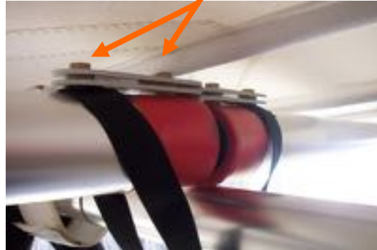
Crossbar center plate bolts looking from front side
